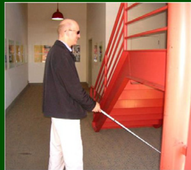
Left: Staircase without cane-detectable barrier. Right: Angled structural element.
