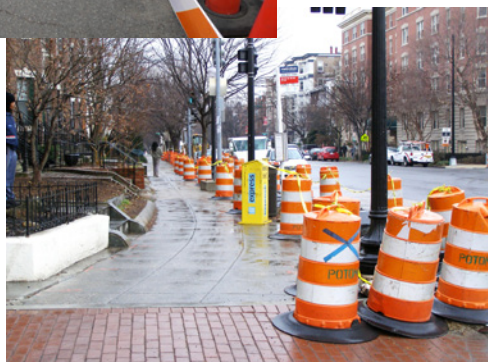
Right: An inaccessible non-continuous barrier that is not cane-detectable.
