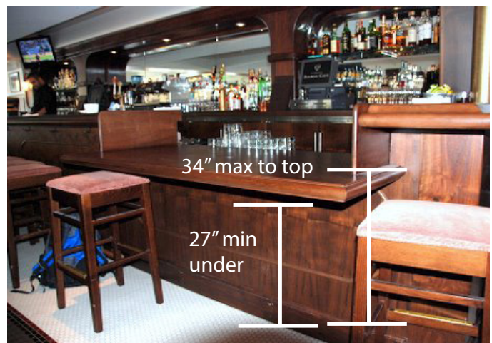
Accessible bar (upper) and bar section (lower): The bar tops are at 34" from the finished floor with the required 27" knee clearance below.
