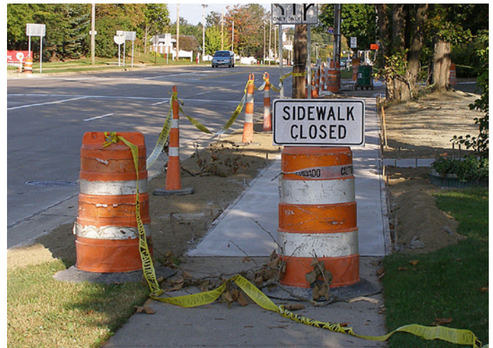
An inaccessible sidewalk closure. No accessible signage for blind pedestrians. Caution tape is not an acceptable barricade.
