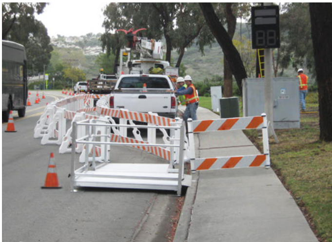
An accessible sidewalk closure and alternate route.
