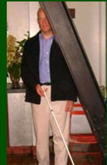
Left: Staircase without cane-detectable barrier. Right: Angled structural element.
