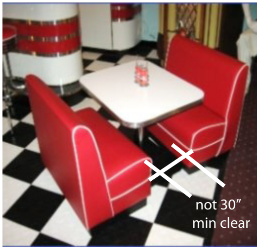
Inaccessible Table: Though this table may have the required measurements for table top height and knee clearance, the fixed bench seating does not allow for someone using a wheelchair to pull up to the table, as there is not a minimum 30" clearance between the benches.
